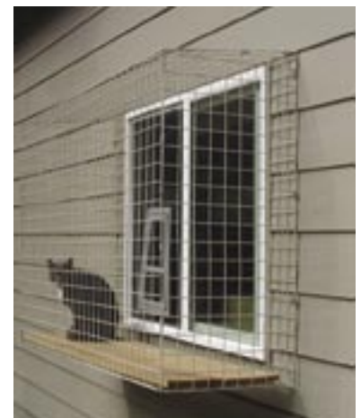
A simple wire mesh enclosure built around a window.
